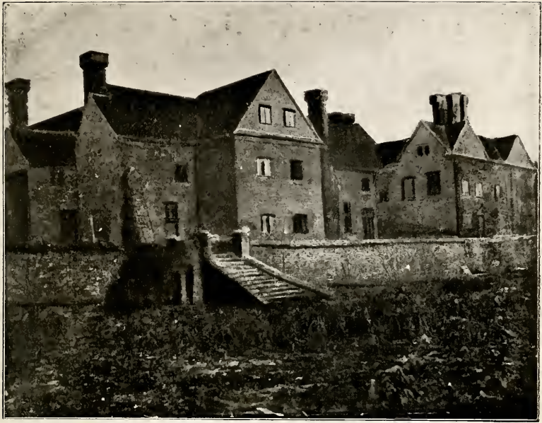
UFTON COURT, BERKSHIRE.
