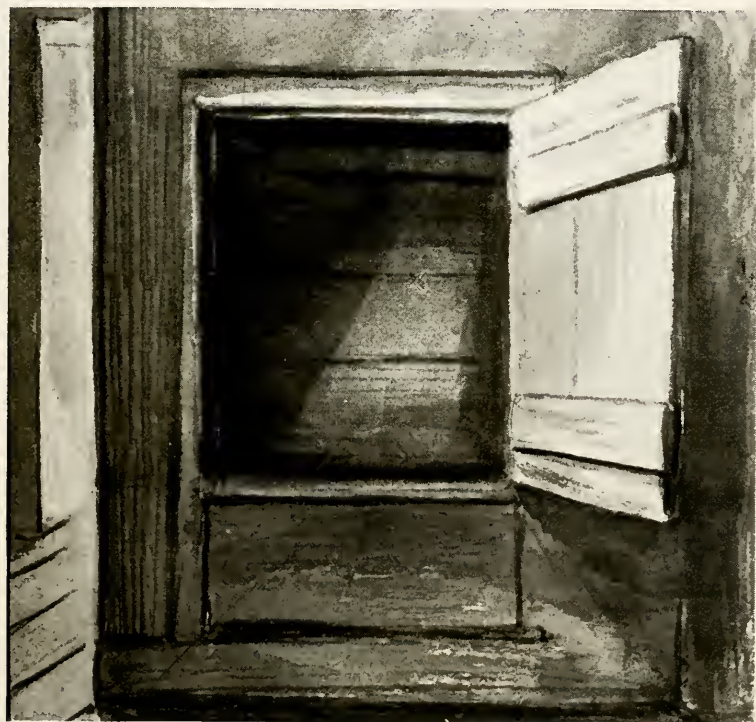
ENTRANCE TO "PRIEST'S HOLE," THE UPPER HOUSE, MADLEY, SHROPSHIRE.
