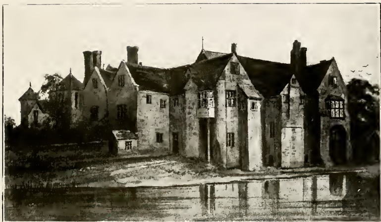
MADELEY COURT, SHROPSHIRE.
