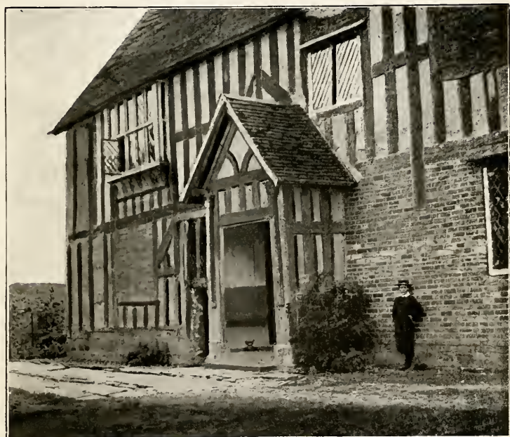
ENTRANCE, HUDDINGTON COURT.
