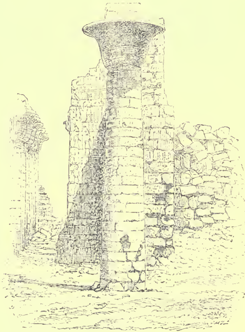
FIG. 130.—Column in the court of the Bubastides, at Karnak.
