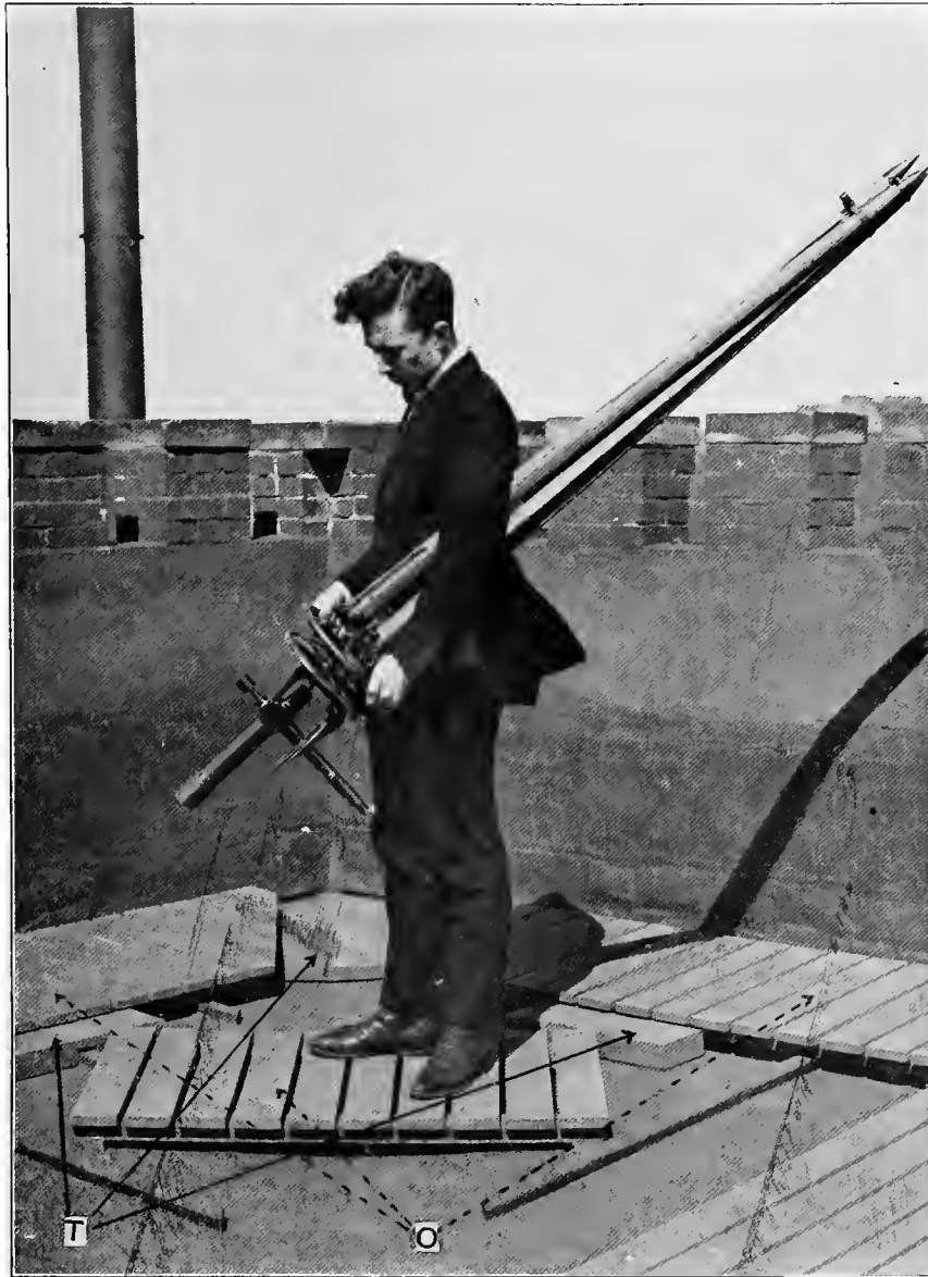
FIG. 38.—Proper method of carrying theodolite, and insulation of theodolite stand ( T ) from observation platform ( O ).
