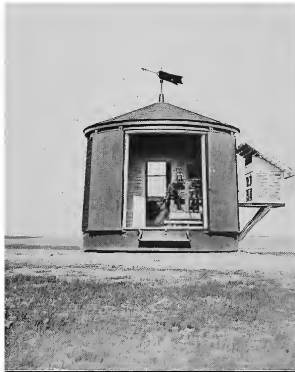
FIG. 3.—Close view of kite-reel house at Ellendale Aerological Station.
